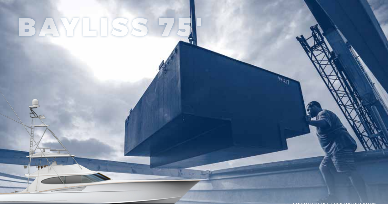
FORWARD FUEL TANK INSTALLATION
